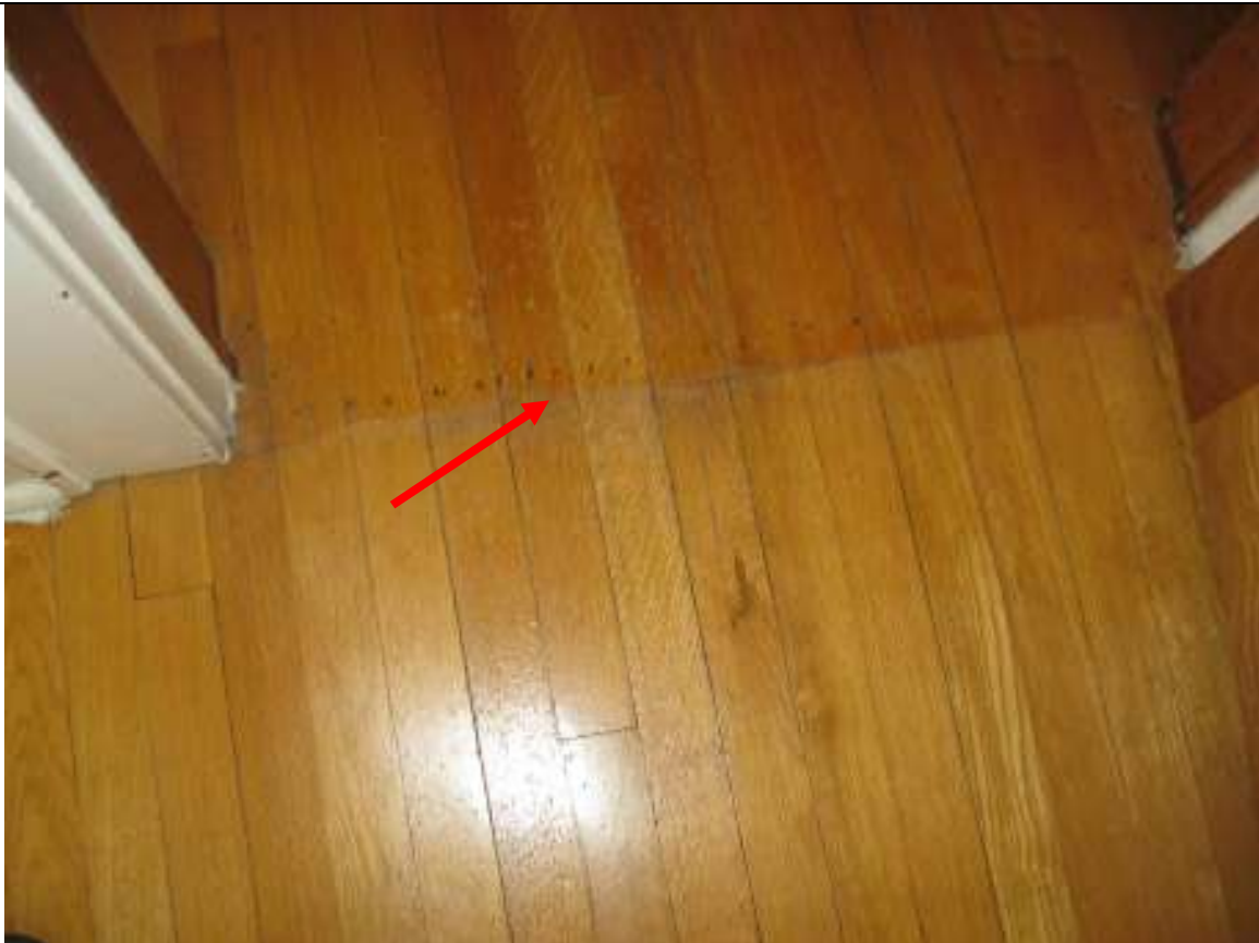
I ST251W0 Street Town Client Image # 20 Hard wood floor on second floor, finished amateurishly
